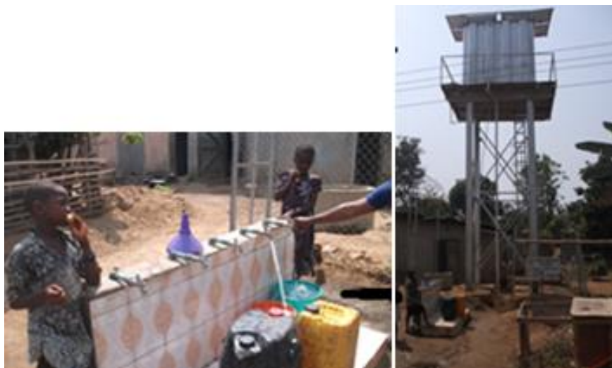
Plate 1. One of the solar-powered water supply outlets in Ondo State, Nigeria
