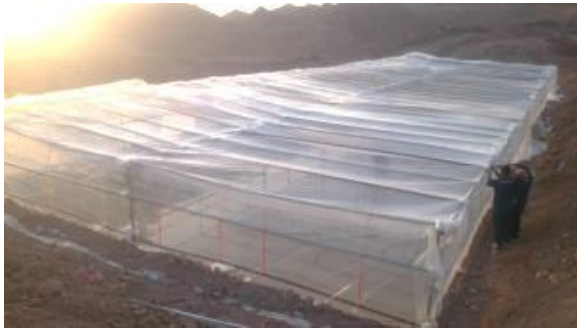
Fig. 3. New HDH based on seawater greenhouse, Naft e Sefid, Shushtar, Khuzestan, Iran, 2019.
